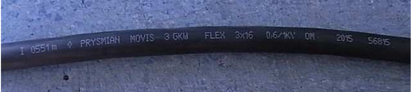
CABLE MARKING : PRYSMIAN MOVIS 3 GKW FLEX 3X16 0,6/1 KV OM 2015 I METER MARKING
