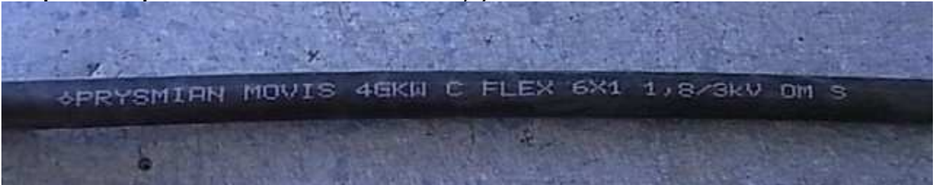
CABLE MARKING : PRYSMIAN MOVIS 4GKW C FLEX 6X1 1,8/3 KV OM S 2015 56816 I METER MARKING
